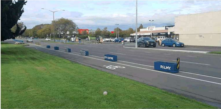
Figure 2: Main Street Temporary Separated Cycle Way
