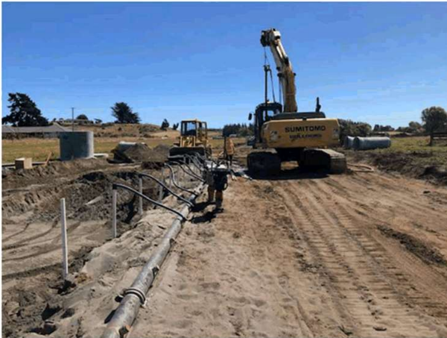
Photo: Fitzherbert Avenue Construction - Heavy storm water pipes and manholes being constructed underground. Dewatering taking place.
